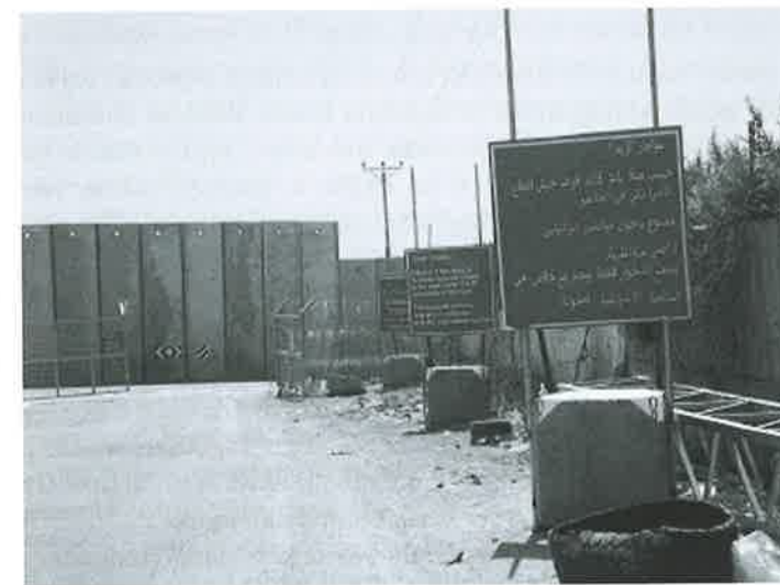
Figure 17.2 Concrete wall separating Israel from Palestine Bakka-El-Garbia, Israel
